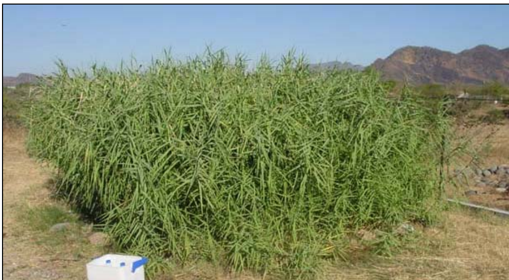
Figure 1 – Pilot scale horizontal subsurface flow reed bed system realized in Nacaome
